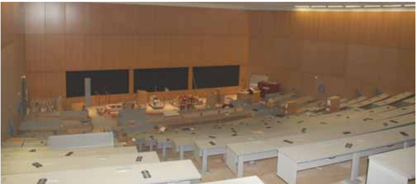
The John W. Lachman Auditorium — A work in progress.
